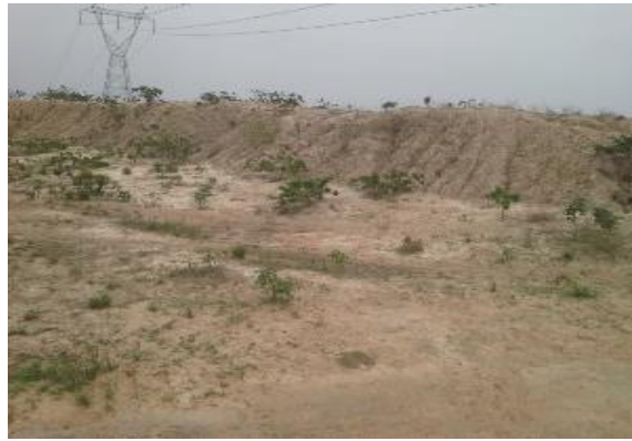
Figure 11: Earth bund fencing within perimeter of Dawa Industrial Park to ward off Cattle and encroachers
