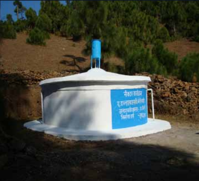
Communities planned and constructed their water supply systems
