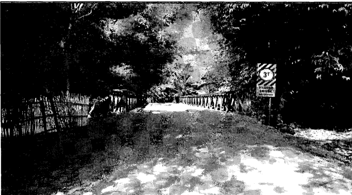
Existing Bailey Bridge (30.35 Lm.) for Replacement Km. 193 + 859
