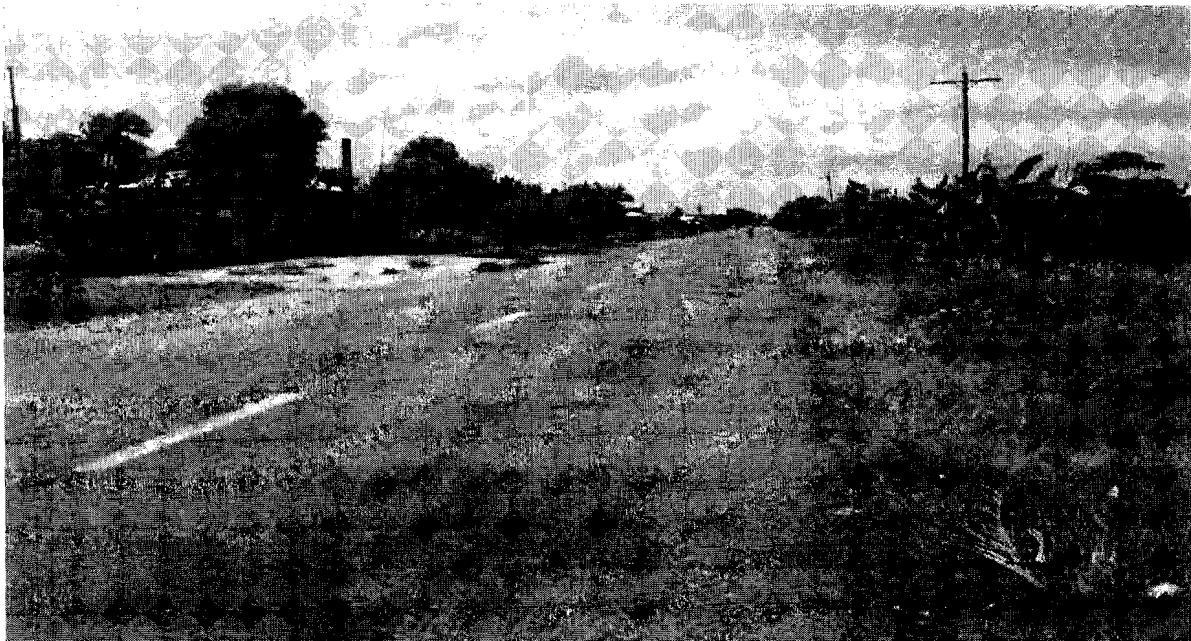
Existing Asphalt Paved Section @ Km. 142 + 000 Brgy. Sta. Brigida
