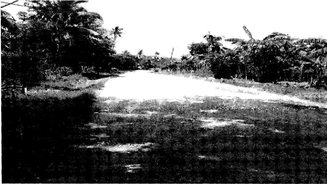
Existing Road Condition (Gravel Section) @ Km. 154 + 900 Brgy. Teresita
