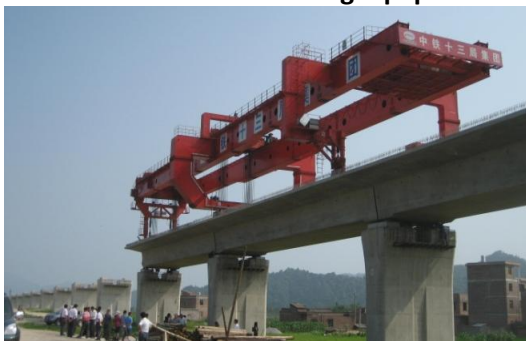
Picture 2. Beam Launching Equipment
