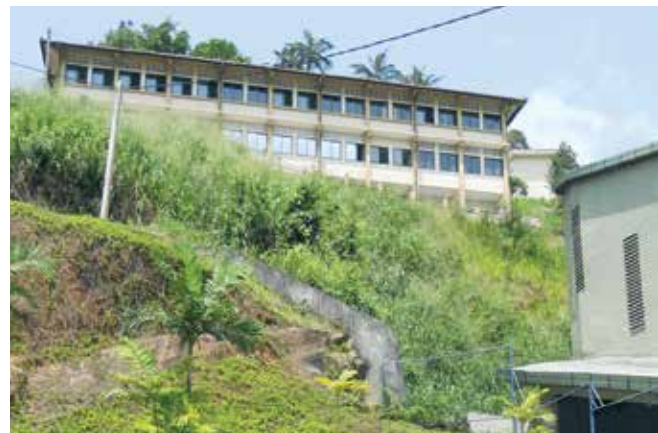
Slope stabilization in schools, Kandy, Sri Lanka Photo by: Suranga Kahandawa
