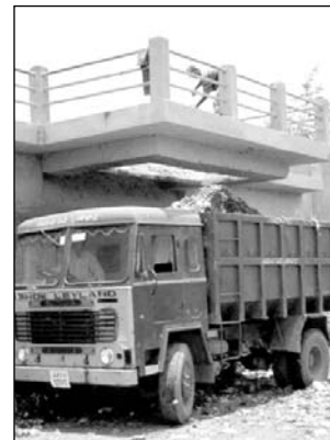
This transfer station has split levels for direct transfer of waste from a small vehicle to a large vehicle.
