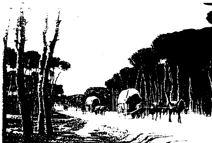
Figure 4-5: The passage of the Damascus road through the Southern Pine Forest during the 1800's. Note that the carriageway has been levelled up and is much higher than the surrounding ground.
