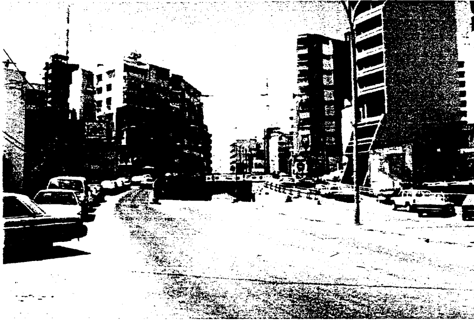
Plate 6-1: Sassine Square looking to the North
