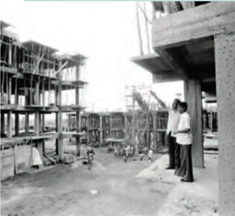
India: HDFC-financed housing units under construction, 1980.
