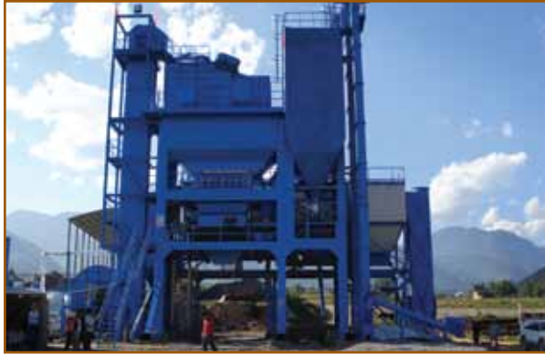
Modern Asphalt Plant on BaoLong Expressway in Yunnan Province, China
