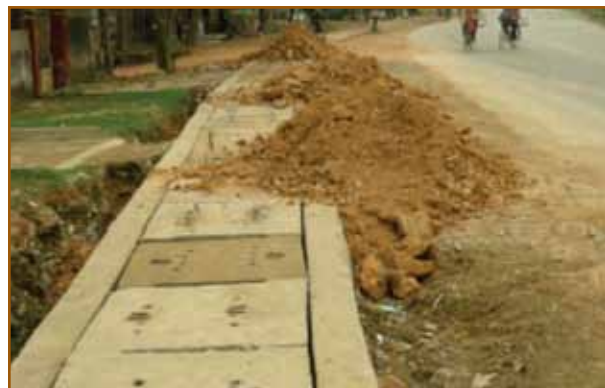
Concrete Drainage Ditch in Urban Area In Vietnam
