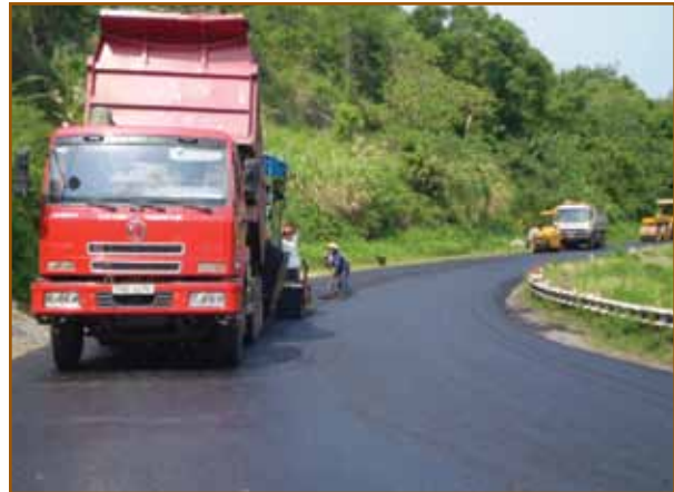
Paving of Binder Course on National Road in Vietnam
