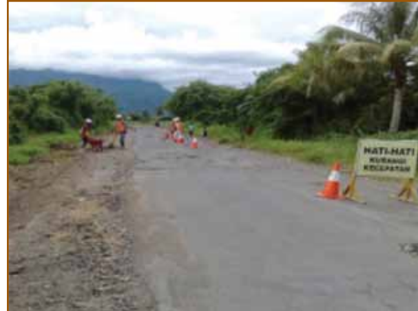
Routine Maintenance Work on a Rural Road in Indonesia
