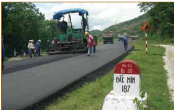
Old Paver in Use on NH26 Rehabilitation Project in Vietnam
