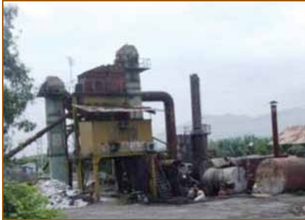
Asphalt Mixing Plant Producing in Poor Conditions in Vietnam
