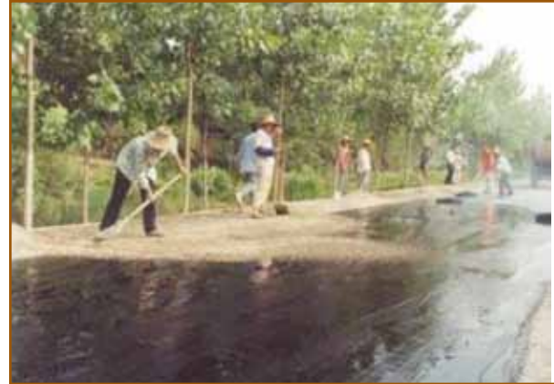
High Labor Intensity in Surface Dressing on County Road in Hubei Province, China
