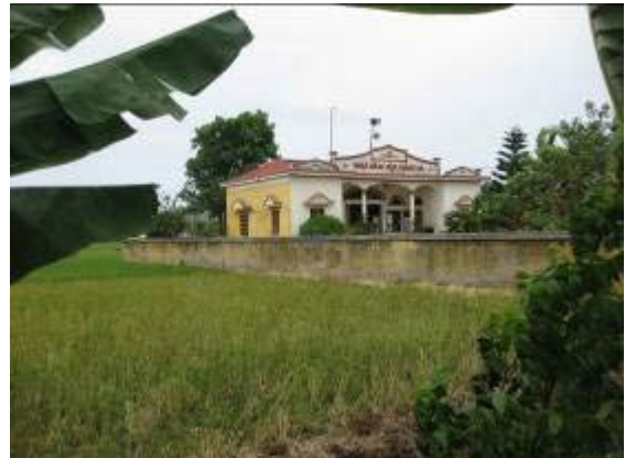
Culture house outside resettlement site, possibly affected by building work with noise, dust, visual impacts
