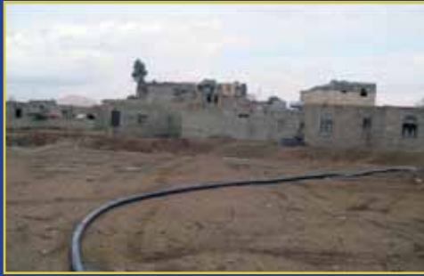
Disposal of sewage in Houd Sana'a
