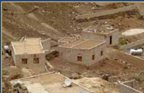
Steep slopes & danger of land slides in Sneina
