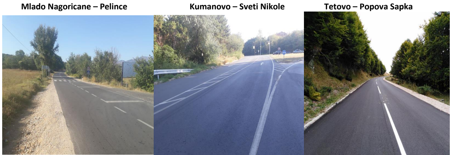
Figure 3: Road segments after rehabilitation
