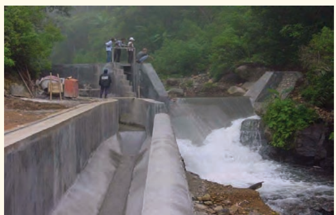
El Bote, a 930-kW hydropower project located in Nicaragua's central highlands, delivers power to 2,700 rural residents.
