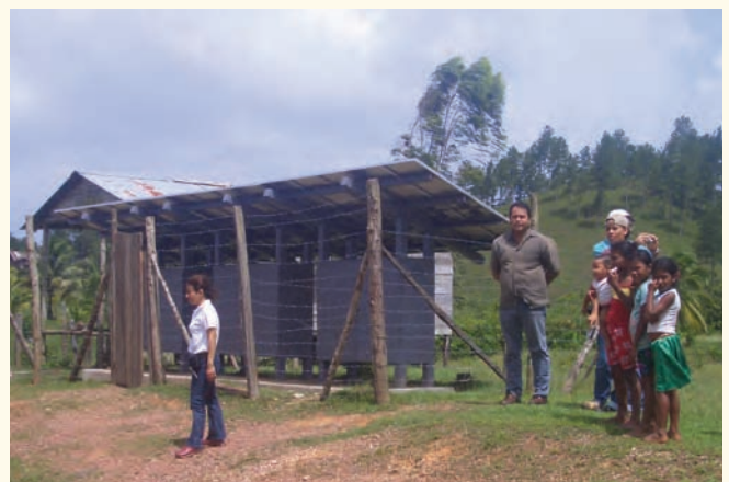
In Nicaragua's remote Atlantic Zone, 350 families benefit from 2-kW capacity, solar battery charging stations installed by the Offgrid Rural Electrification Project (PERZA).
