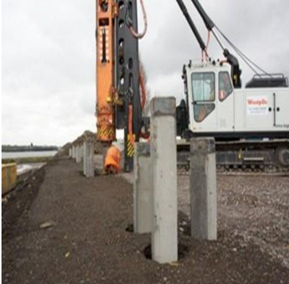
Concrete driven piles
