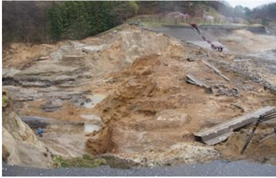
Earthquake (Fujinuma Dam, 2011 earthquake)
