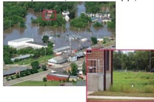
Flood (pump station inundation)
