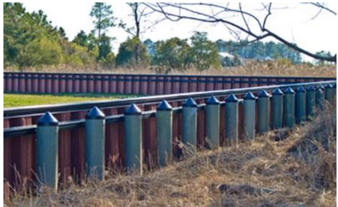
Steel sheet piling
