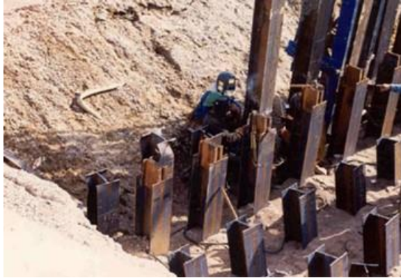
Steel H or pipe piles
