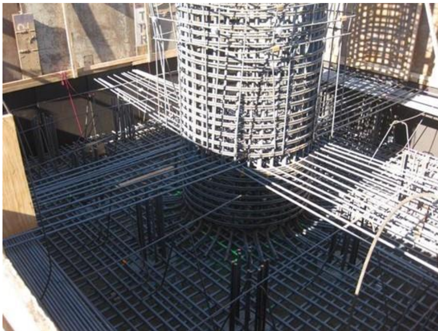
Figure 113. Ductile detailing of concrete columns
