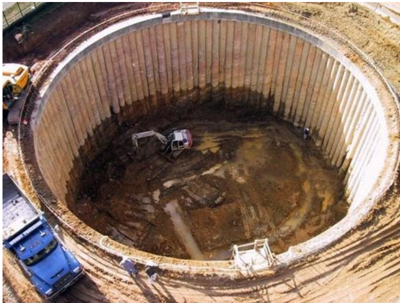
Figure 71. Secant piles
