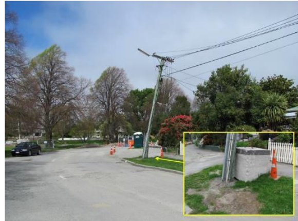
Liquefaction (Christchurch Earthquake, 2011)
