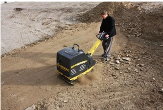
Vibro compaction of a gravel road
