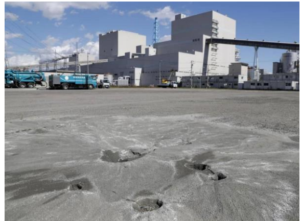
Liquefaction (Hokkaido Earthquake, Japan, 2018)
