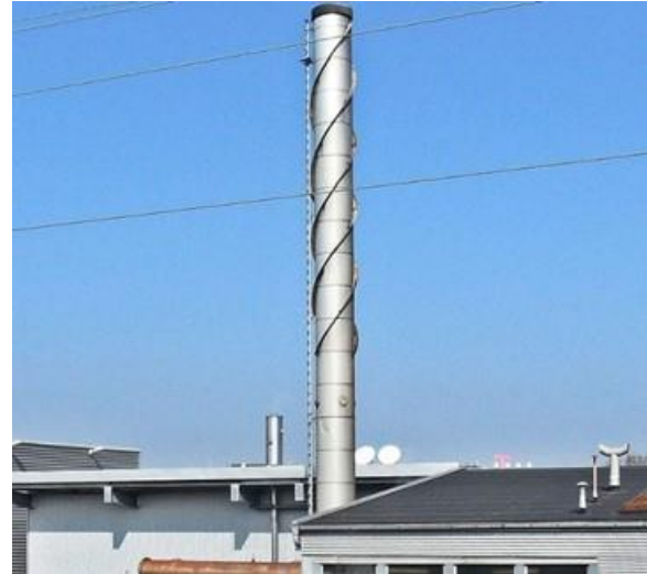
Helical strake for crosswind
