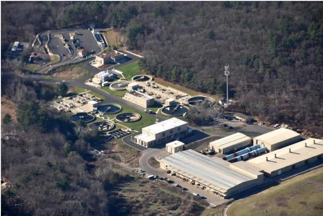
Figure 72. Wastewater treatment plant, Massachusetts, USA
