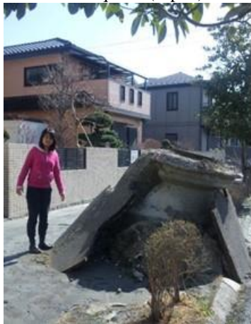
Liquefaction, sewage manhole (Japan)
