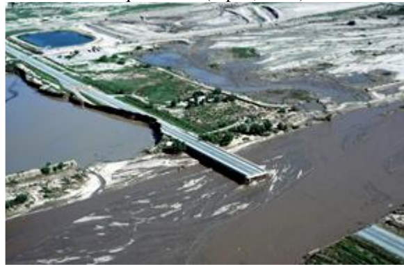
Flood (Arizona, USA, 2017)
