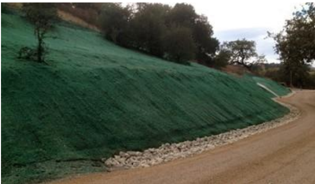
Erosion control by hydroseeding
