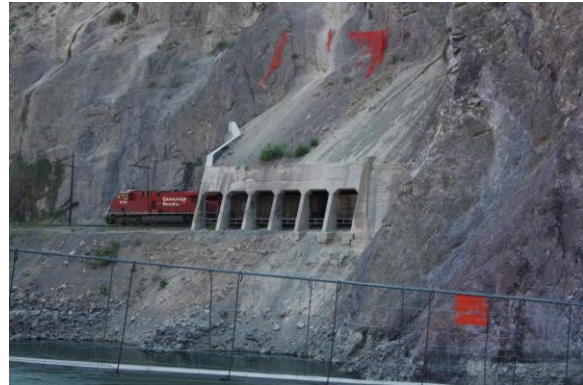
Concrete-frame rockshed (Canada)
