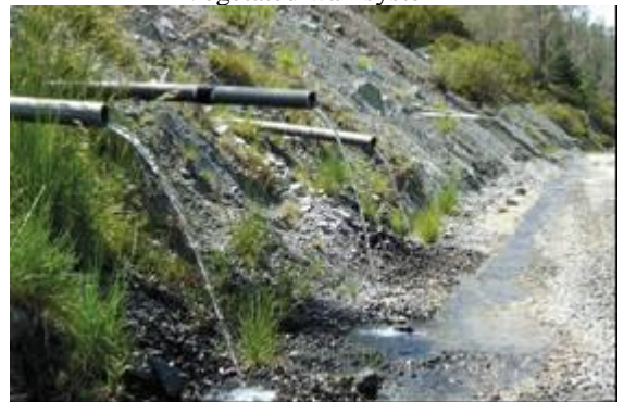
Drainpipes (installation example)
