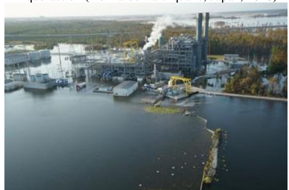
Flood (aftermath of Hurricane Florence, 2018)
