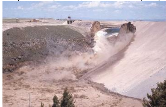
Flooding (Teton Dam, Idaho, USA, 1976)
