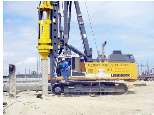
Concrete pile addition
