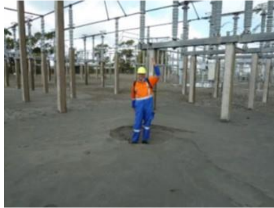
Liquefaction (Christchurch Earthquake)
