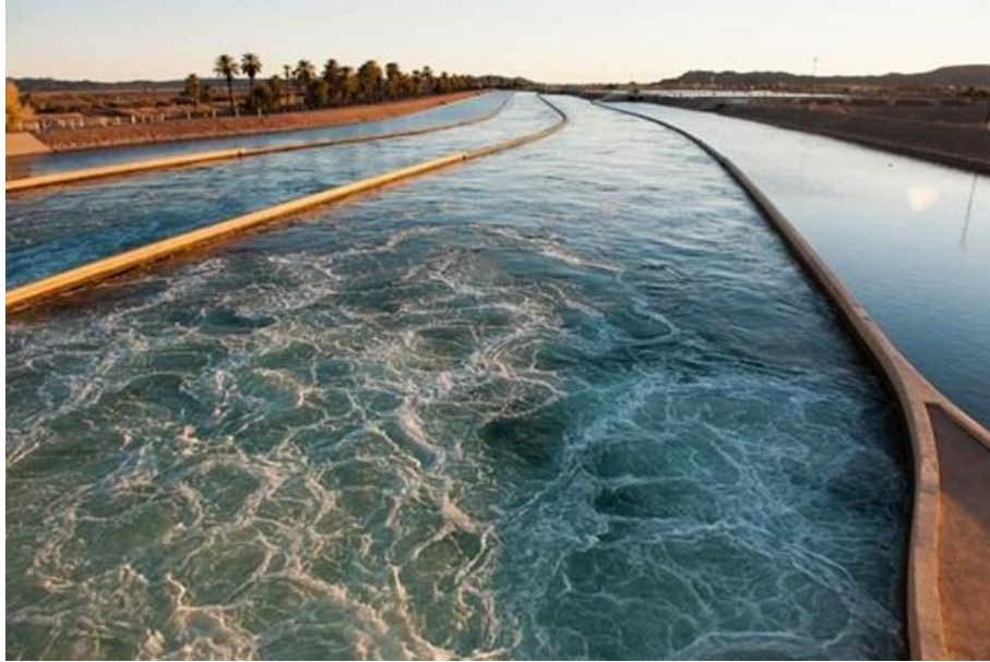
Figure 93. Water canal (Arizona and California, USA)
