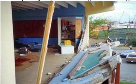
Wind (wall wind out-of-plane damage)
