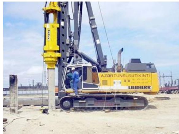
Prestressed driven piles
