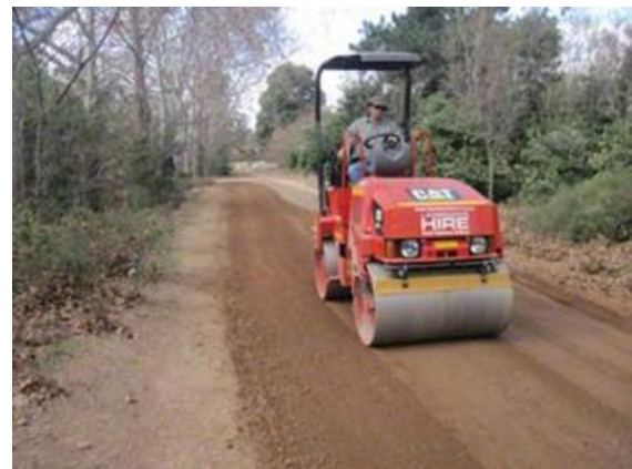
Dynamic compaction of a gravel road
