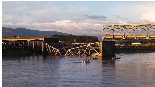
Earthquake truss failure
