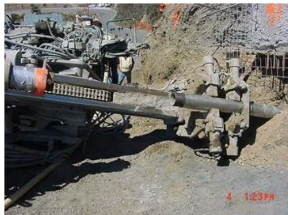
Soil nails, tieback anchors
