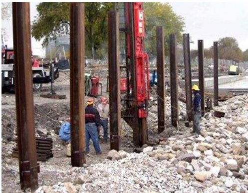
Steel pile addition
