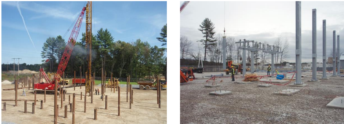
Figure 35. Example of liquefaction mitigation
