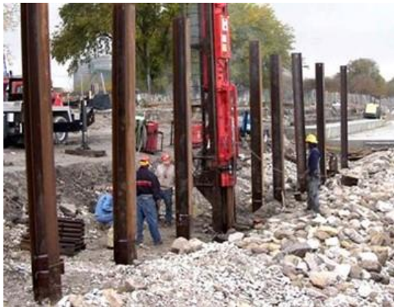
Steel H driven piles
