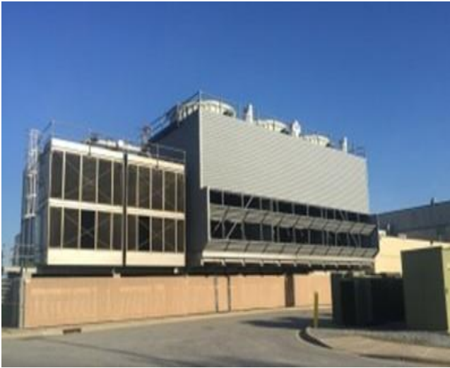
Braced cooling tower support structure
