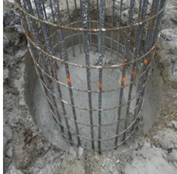
Concrete drilled piles
