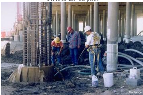
Cast-in-drilled-hole (CIDH) pile
