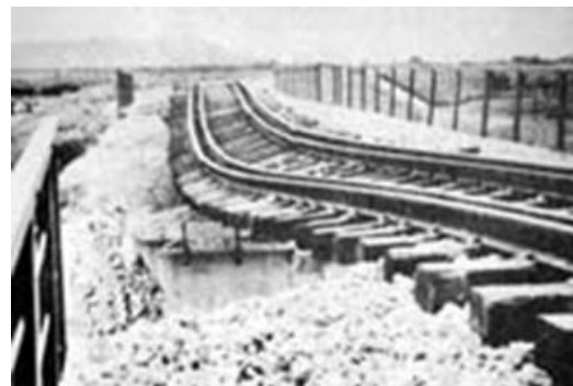
Liquefaction (soil subsidence and deformation)
