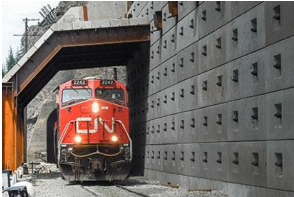
Steel-frame Rockshed (Canada)
