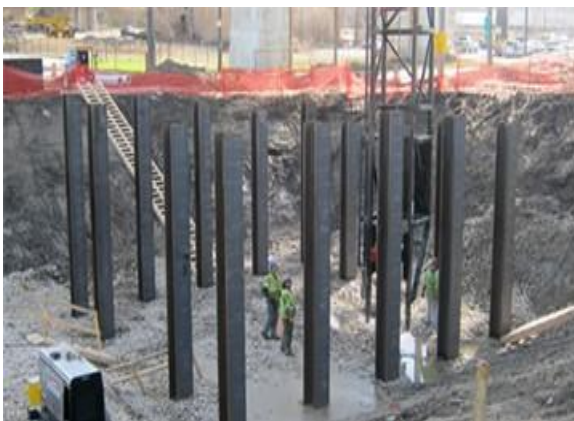
Steel driven piles
