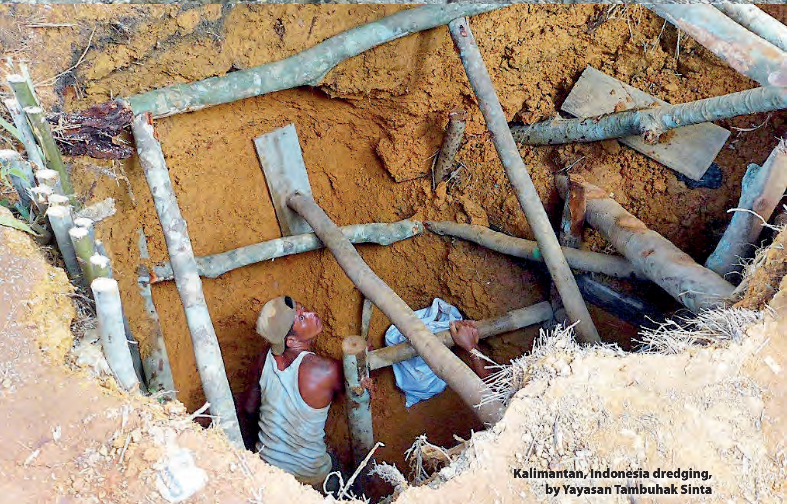
Dredging in Kalimantan Credit: Yayasan Tambuhak Sinta
