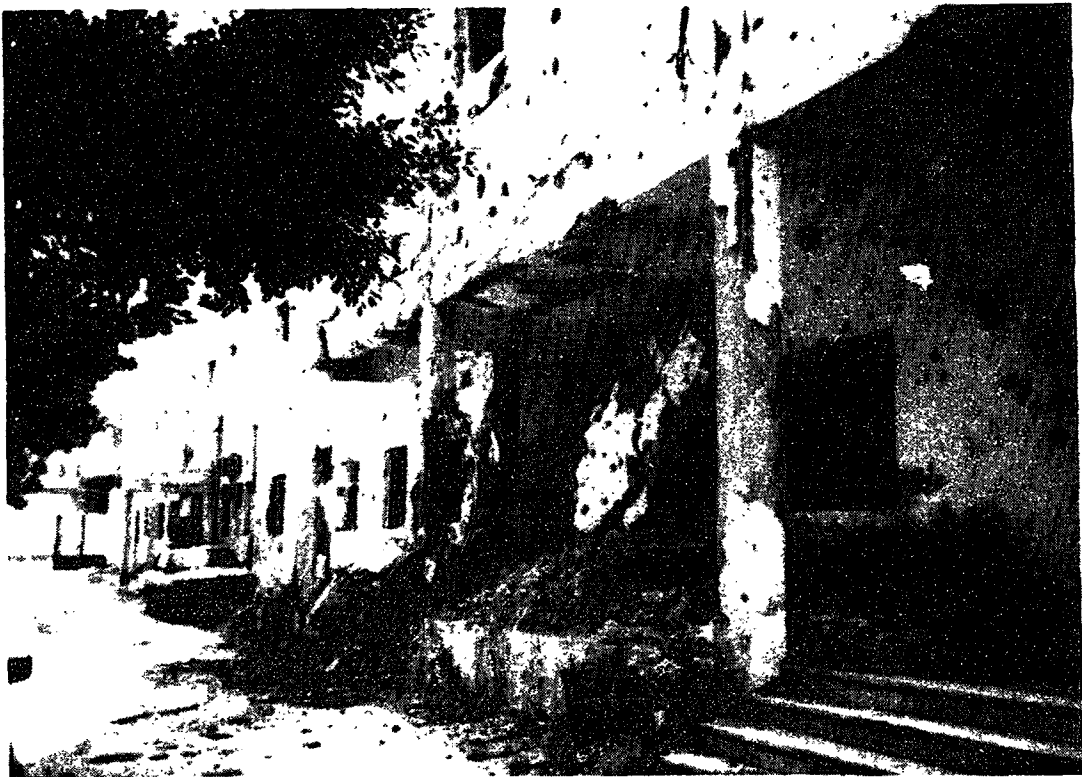
Beirut: Damage to Quarantine Hospital
