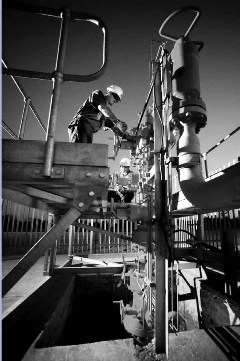
The gas pipeline between Mozambique and South Africa was the first cross-border pipeline in Sub-Saharan Africa. The project was guaranteed by MIGA and the World Bank to mitigate political risks. Photo courtesy of Sasol.
