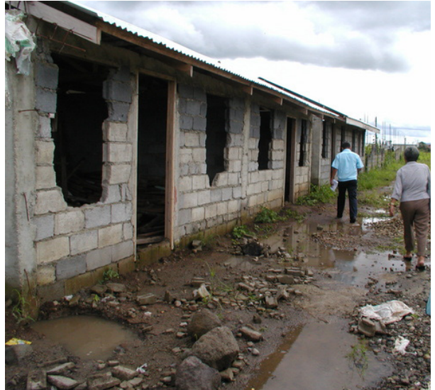
Photo: Urban revitalization works during the UPSURGE project the World Bank.
