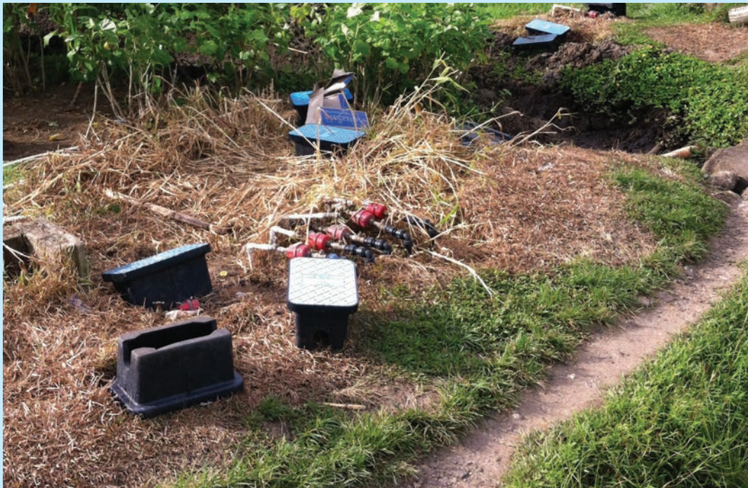
FIGURE 3.2: WATER METERS AT THE EDGE OF A SETTLEMENT IN SUVA
