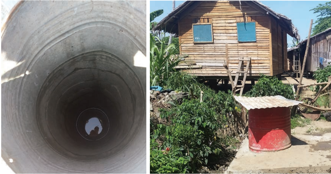
FIGURE 3.8: SHALLOW WELL LINED WITH DRUMS IN BURNS CREEK NEAR HONIARA
