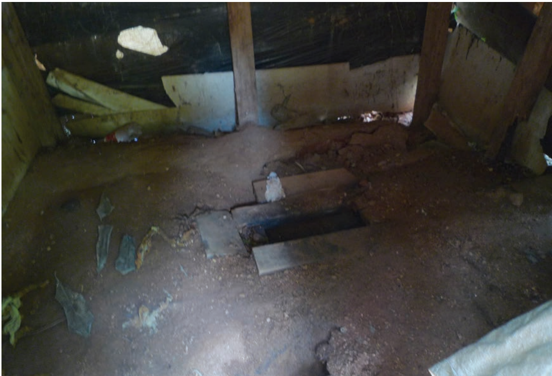
FIGURE 3.4: INTERIOR OF A TYPICAL DRY PIT TOILET IN PNG
