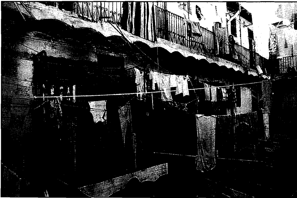
Interior of an over-densified and dilapidated oukala, which has been demolished.
