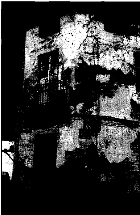
Exterior of a dilapidated oukala.
