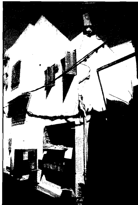
Building rehabilitation by owner occupant with income generated by the ground floor commercial use.
