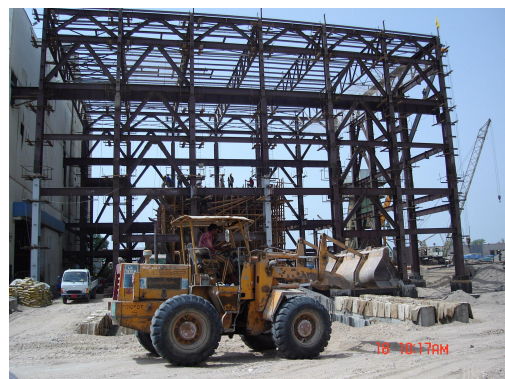
Figure-3.2.13 New 6 th Generator under Construction
