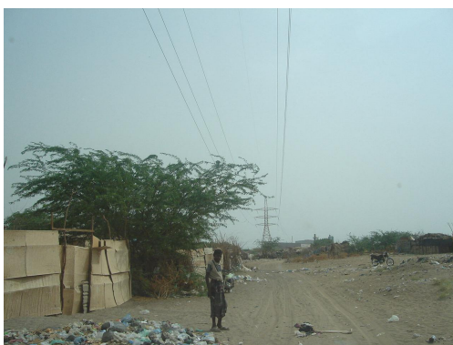
Figure-4.3.8 Some Squatters Found within ROW of Existing
