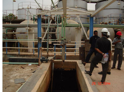
Figure-4.2.6 Water Sample Collection from Boiler Blow Down
