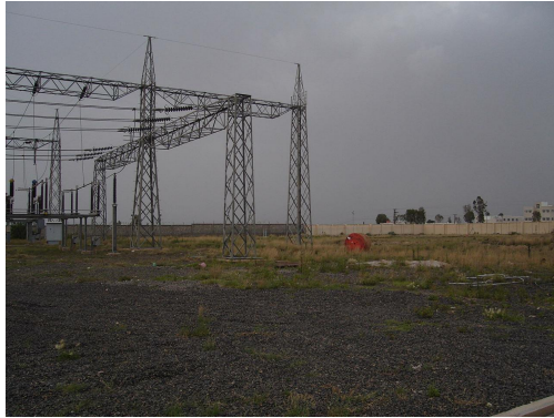
Figure-3.3.6 Space for Expansion of 132 KV Dhamar Substation
