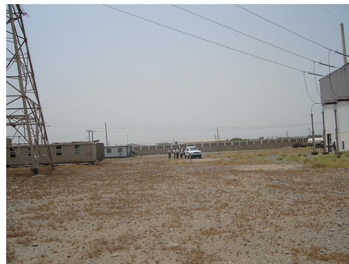
Figure-3.3.3 Space for Expansion of 132 KV Al-Hali Substation
