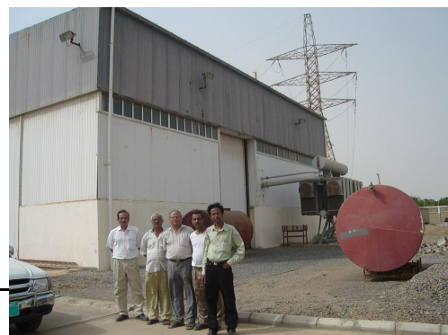
Figure-3.3.2 Existing 132 KV Al-Hali Substation
