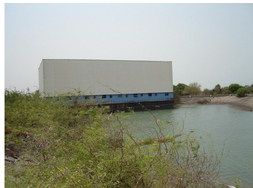
Figure-3.2.6 Cooling Water Intake Pump House
