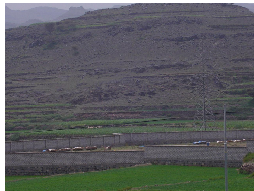
Figure-3.3.7 Site for New 132 KV Yarim Substation
