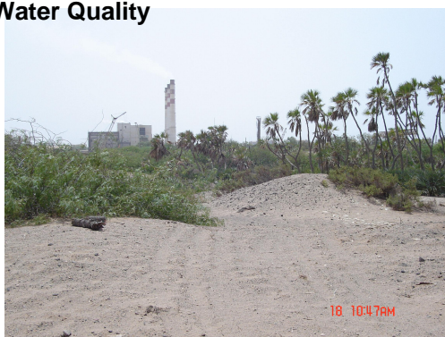
Figure-4.2.2 Landuse on West Side of Al-Hiswa Power Station
