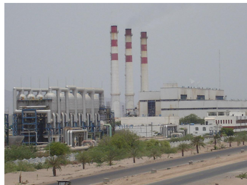
Figure-3.2.2 Al-Hiswa Power Station
