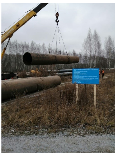
Reconstruction process of water supply of Proletarskiy okrug in Tula
