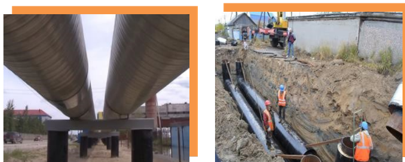
Performing of works on reconstruction of heat networks in Nefteyugansk
