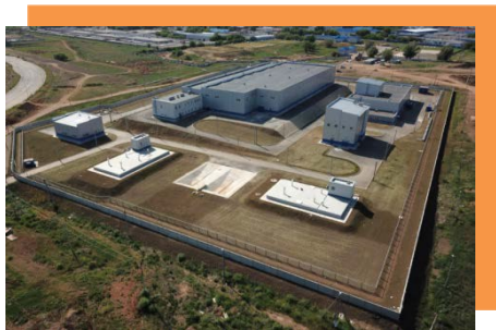
Water treatment plants site of the South-Ural water intake pipeline in Orenburg
