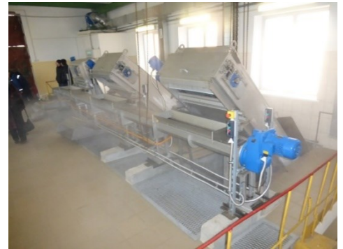
Mechanical wastewater treatment plants: grating and primary radial sump
