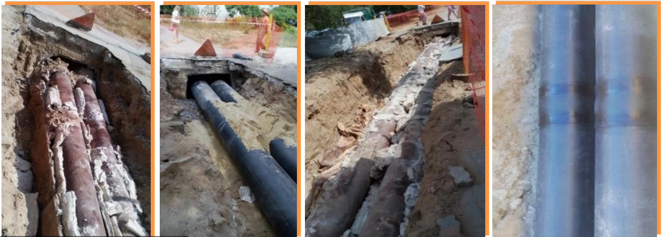
Replacement of pipes of heat pipeline
