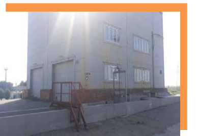
New bar screen building (sewage mechanical treatment facility) of biological treatment plants in Volzhsky
