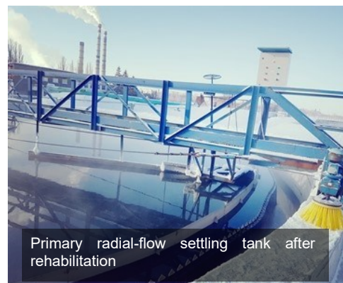
Mechanical wastewater treatment plants: grating and primary radial sump
