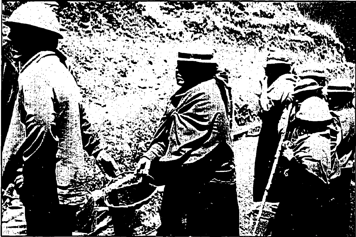
In Peru, female laborers work on a water-diversion scheme, lining a canal that will carry water from the Andes to their village. Such projects are village-based and tend to involve participation from women.
