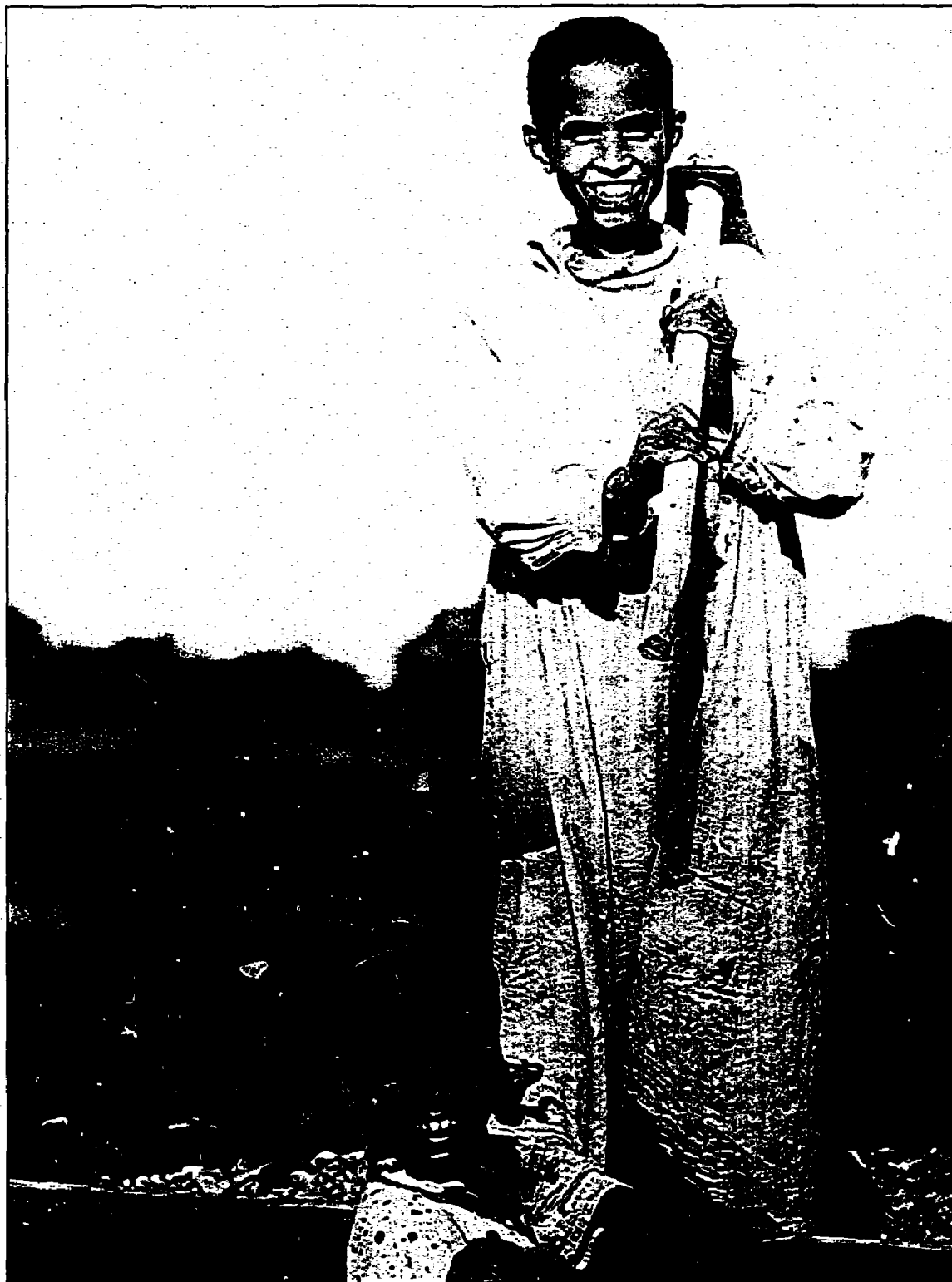
Young workers in Egypt lay drainage pipes in a waterlogged field near their village.
