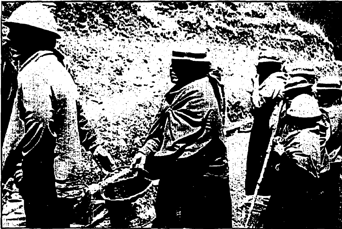
In Peru, female laborers work on a water-diversion scheme, lining a canal that will carry water from the Andes to their village. Such projects are village-based and tend to involve participation from women.
