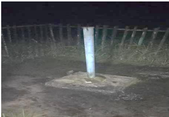
Sharp Pit Disposal in a Rural Health Care Facility
