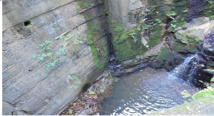
Stilting Basin of Heelpan-Kandura Stream at Ch. 200m
