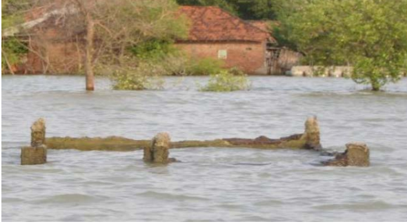
Flooded house in a village in Demak. (Source. Boskalis)
