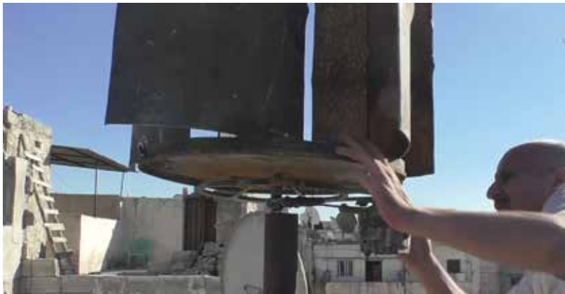
A resident mounts a cut barrel to ensure that it captures wind flow; it is installed on the roof of a building.
