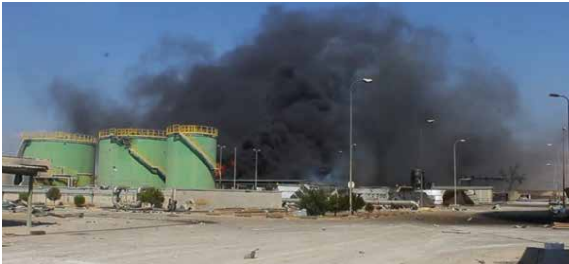
Figure 22: Aleppo Thermal Power Plant Damage (Exterior)
