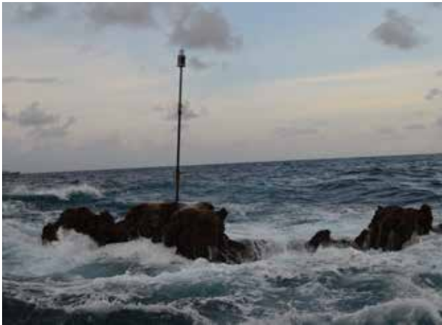
Figure 13. LTE with navigational aid installation.
