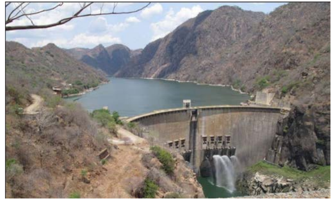
Cahora Bassa Dam
