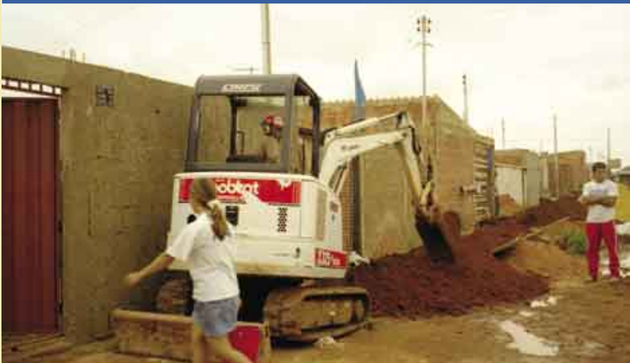
Excavation for the Public Network, Brasilia
