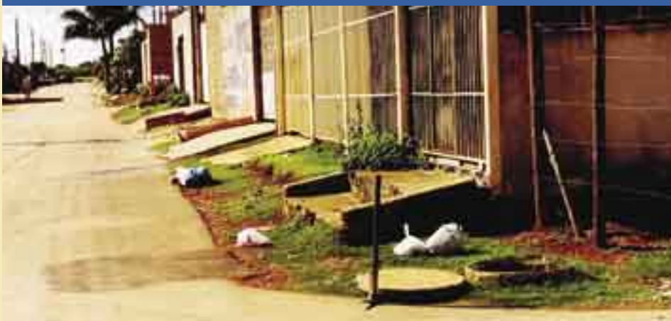
Condominial Box (seen open in the right hand lower corner), Riacho Fundo, Brasilia
