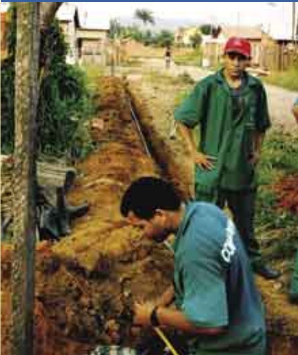
View of Condominial Water Branch, Parauapebas
