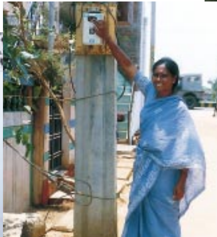
Power being switched on to start the jetpump
