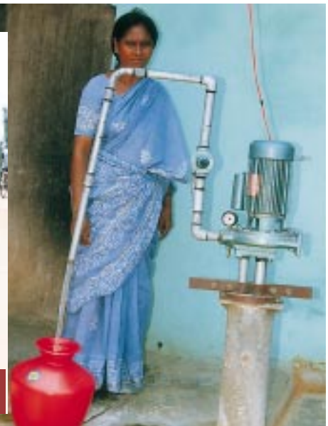
Collecting water from the jetpump
