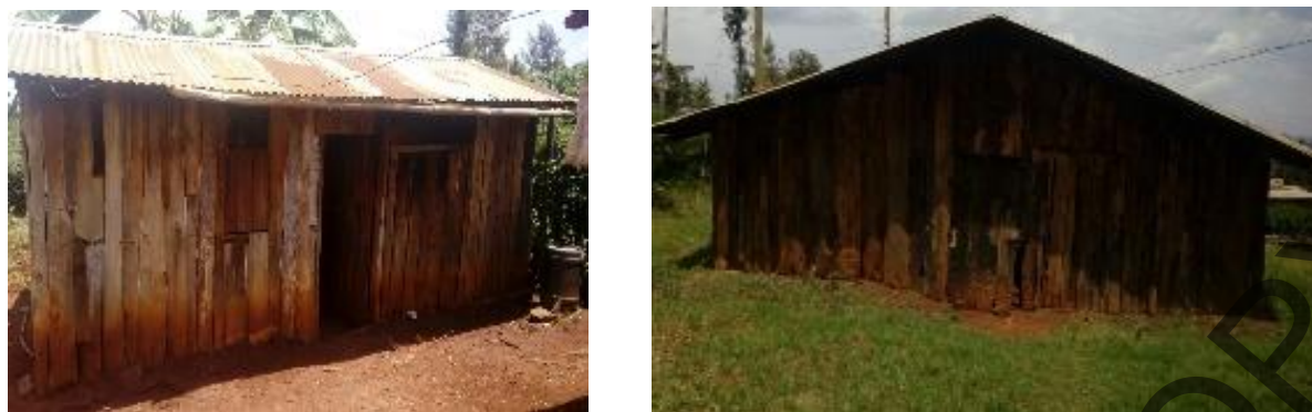
Figure 6-2: Sample photographs of affected structures in the settlement.
