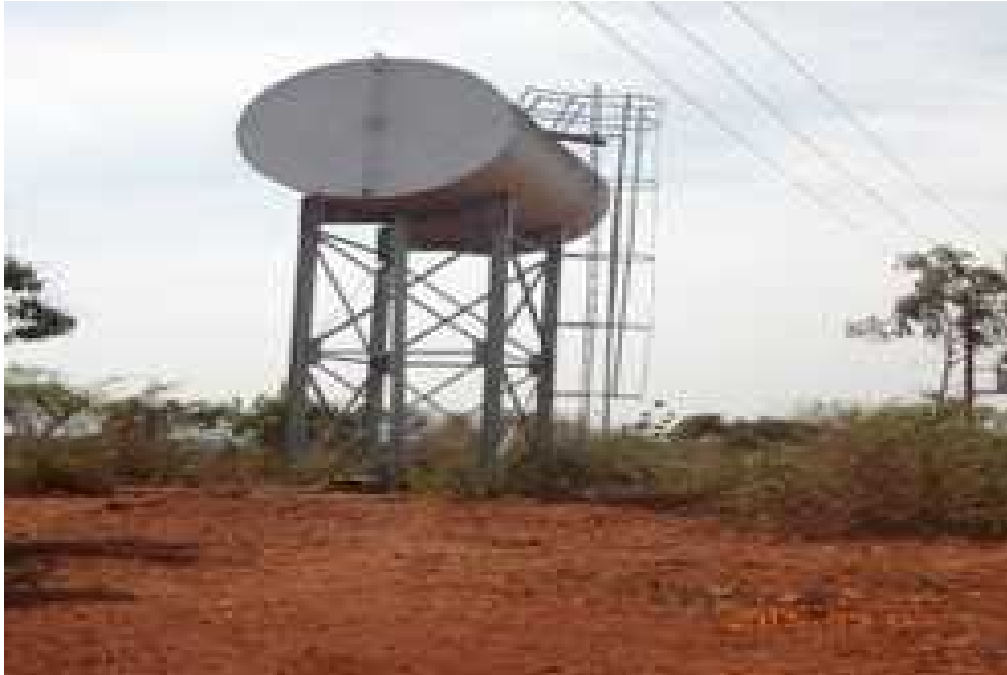
Plate 9: Reservoir 1 at Majanji Parish, Majanji Sub County.
