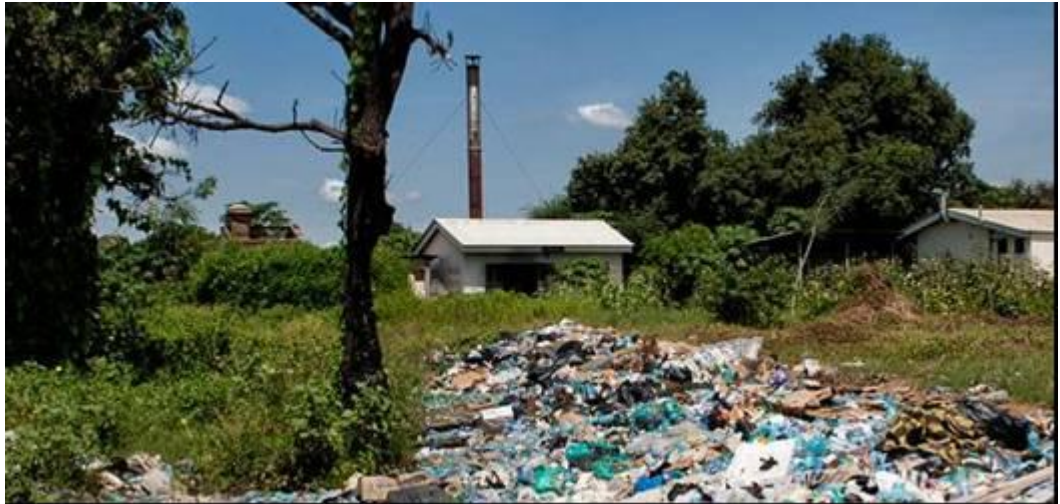
Figure 3-5: Incinerator of the Juba Teaching Hospital
