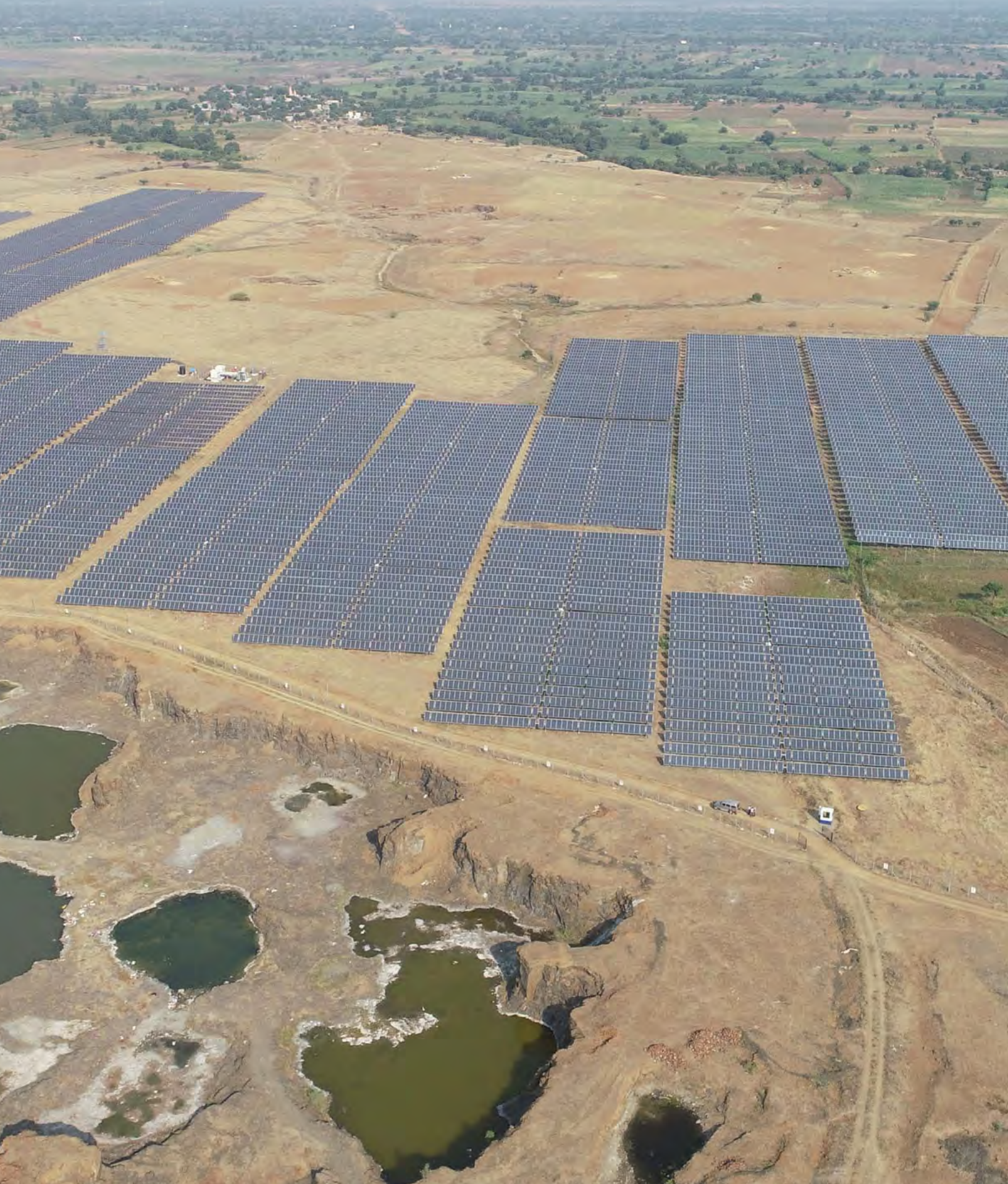
Solar Power Plant, Maharashtra, in state of Maharashtra, India. Photographer: Thomas Lloyd Group, Creative Commons Attribution-Share Alike 4.0 International license.
