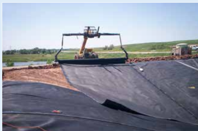
HDPE liner for new landfill cell construction. Photo: © Mike Kleist | Dreamstime.com
