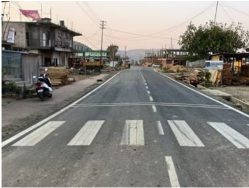
Road Marking at Zotlang Village CZ Road
