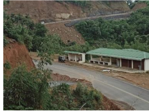
Bazar Shed & Waiting Shed at CC Road
