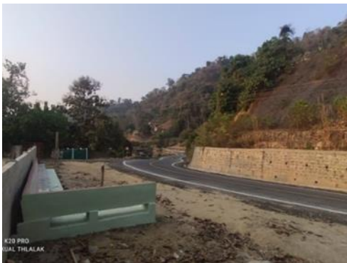
TK Road at Ch: 0+400 Km
