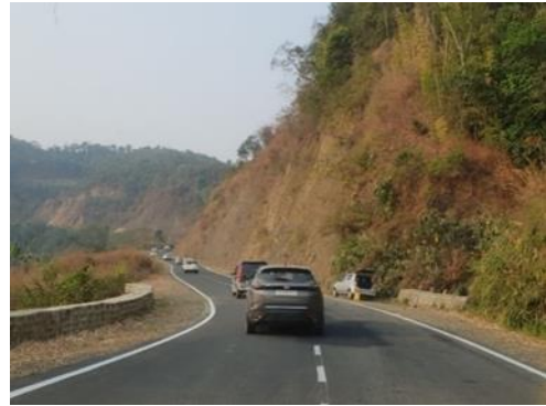
Mualkawi Bypass along CZ Road
