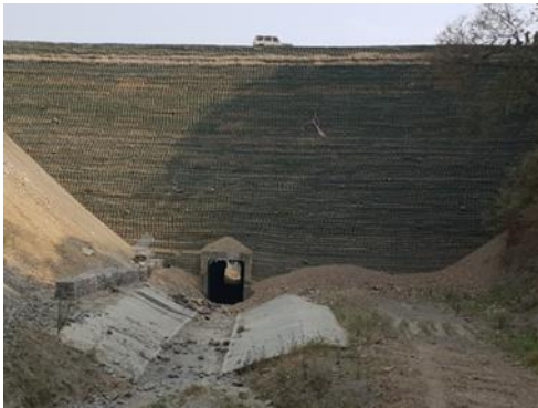
Box Culvert with Geo Cell Embankment at Ch: 21+74
