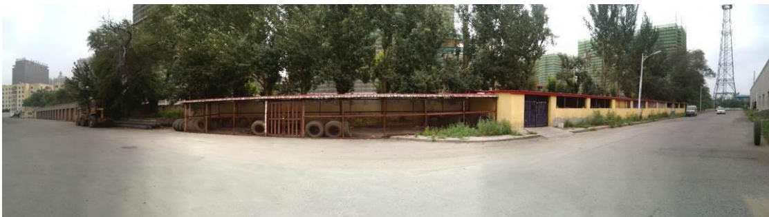
Buildings to be removed (garages and simple warehouse, etc.)
