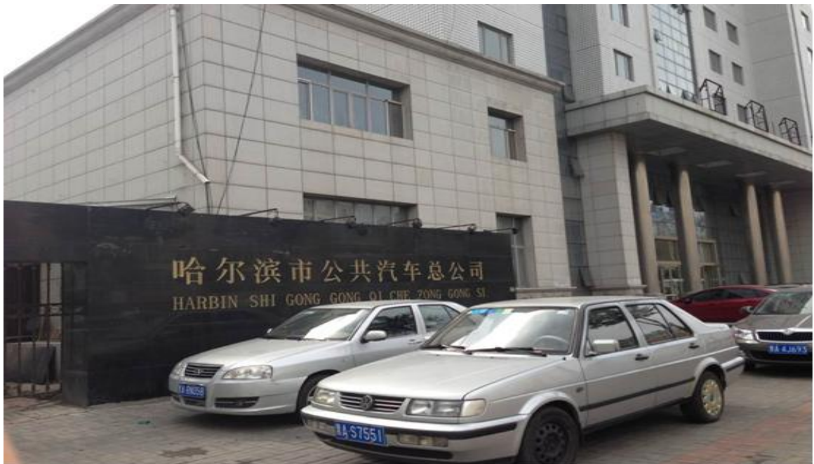
Harbin City Bus Corporation (No.30 at Xiangbin Road )
