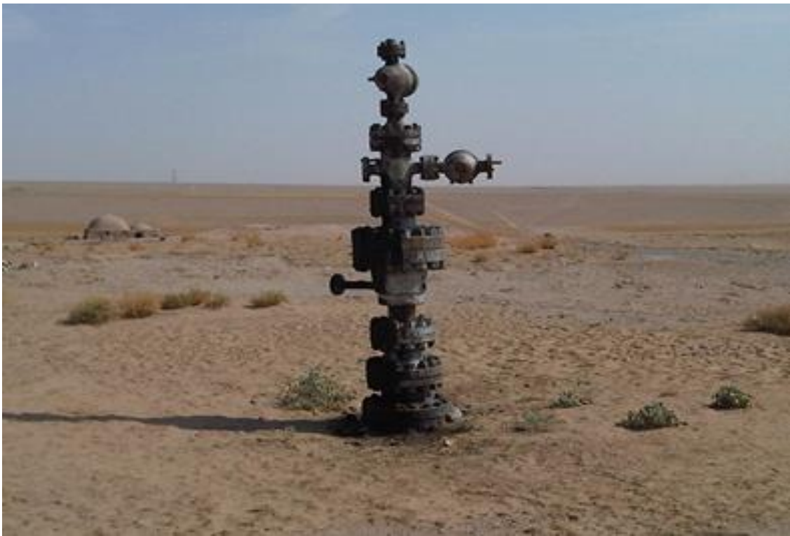
Figure 3- 3 Sheberghan Gas Well
