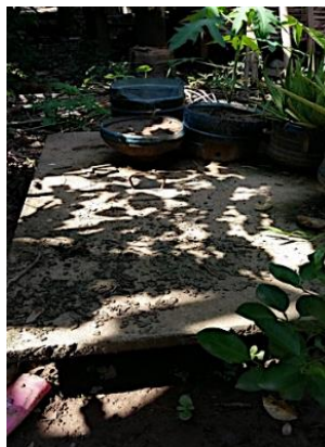
Latrine Tank Seen Above Ground. Source: PSI Research Team
