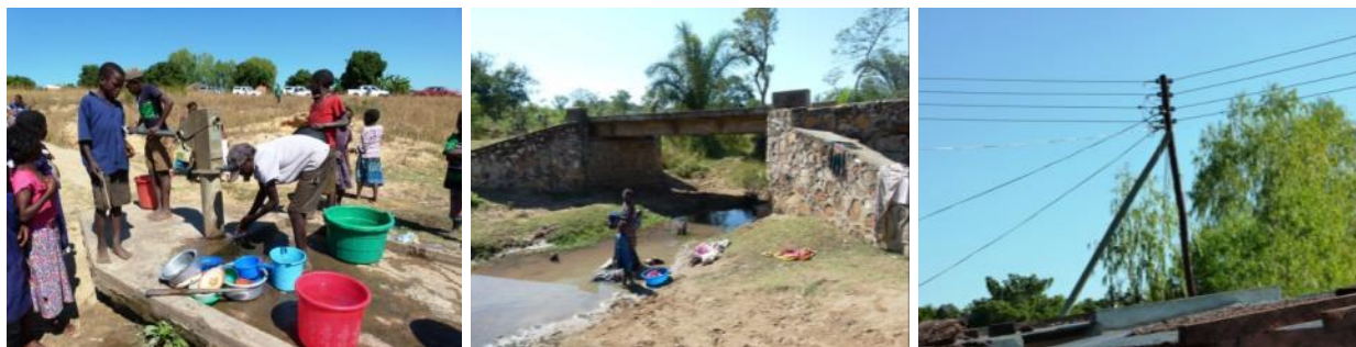
Figure 8: Boreholes, bridges and electricity are crucial infrastructure in the catchment
