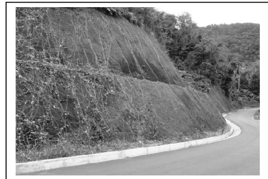
Example of lateral slope stabilization as applied on the rehabilitated road through the Central Forest Reserve
