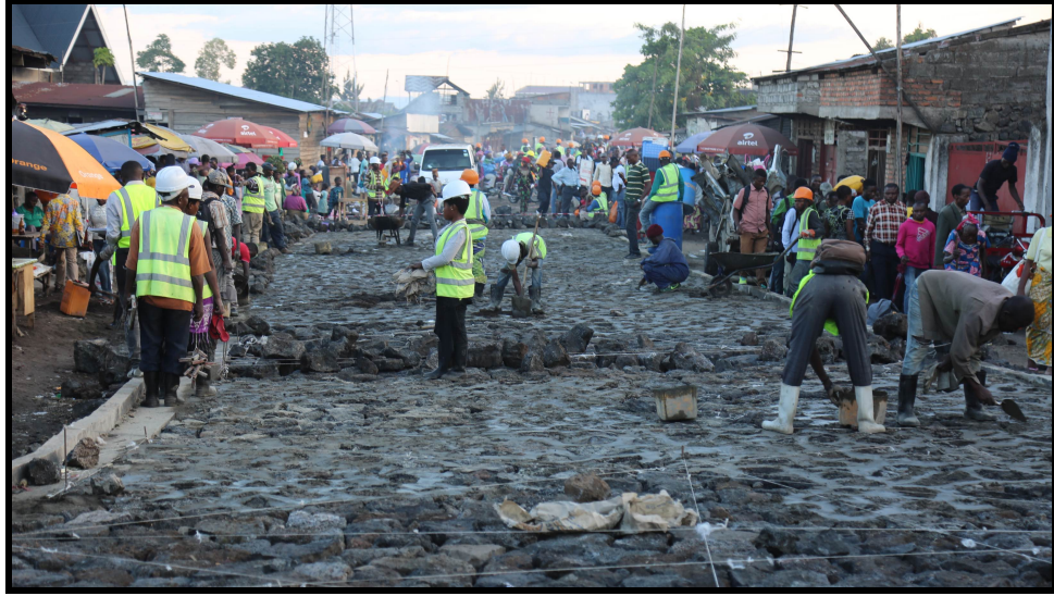
Road maintenance by beneficiaries, Nyabushongo LIPW (Goma, May 2017)
