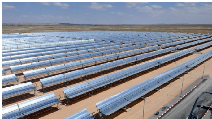
Noor Concentrated Solar Power Plant in Morocco supplies clean energy to millions of beneficiaries. –Dana Smillie/World Bank
