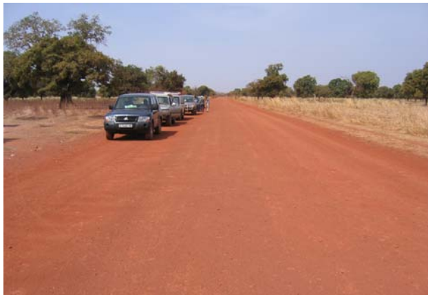
Typical engineered gravel Regional road between Fana and Dioila (R18)
