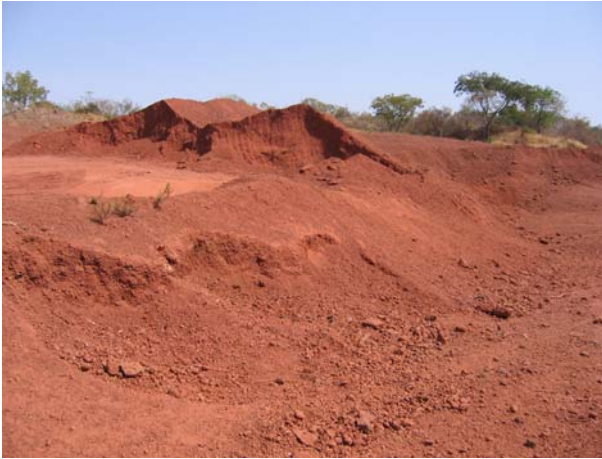
Stock piled, as-dug wearing course material from laterite borrow pit
