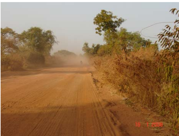
Typical laterite gravel road. Generation of dust is a constant hazard to inhabitants living nearby and their crops as well as posing a serious road safety problem to overtaking motorists
