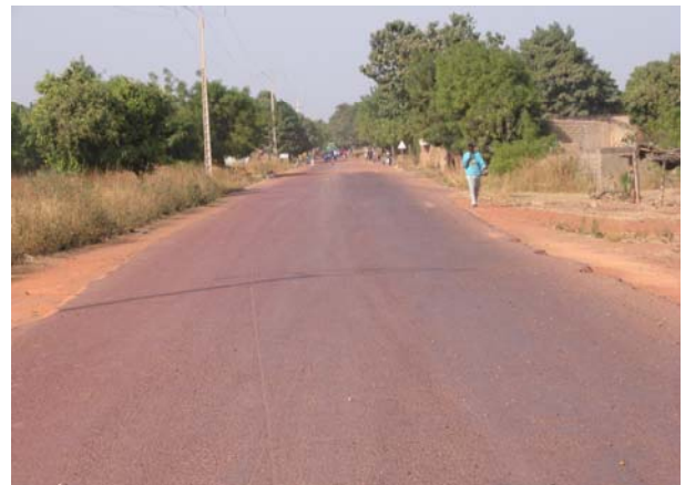
Typical bitumen surfaced National road between Bamako and Koulikoro
