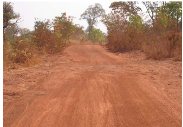
Typical un-engineered, gravel roads in cotton growing area south of Bamako
