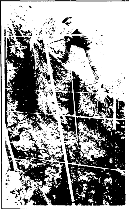
Photo # 15. Malaysia - East - West Highway. Cross section of vetiver hedgerows (photo #14) across road fill embankment. Note overlay lying on original land form (see root - lower right). Vetiver roots have struck through fill into original material - some measure 3.4 meters. Photo credit...P.K.Yoon
