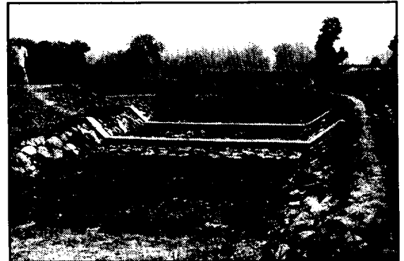
Photo #8. India. Phulbani District, Orissa. Vetiver used for spillway stabilization - note vetiver has been heavily grazed. Photo Credit... R.G.Grimshaw
