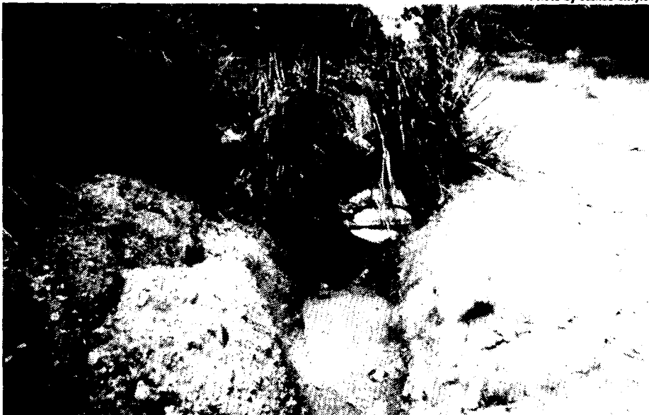
Photo 3. Roadside stabilization with vetiver grass includes protecting culverts from scouring. Photo taken at one of Dr. Yoon's demonstration areas.
