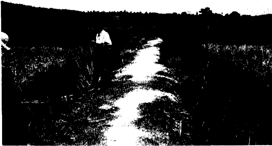
Photo # 12. Vetiver planted to bind earth banks which were constructed to prevent the brackish water from flowing into the fields at the Pikun Thong Royal Development Study Centre. Photo credit: Dr. Sumet Tantivejkul
