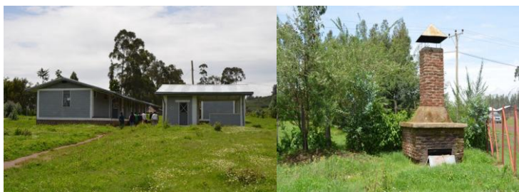
Picture set 3: Health center and health center incinerator
