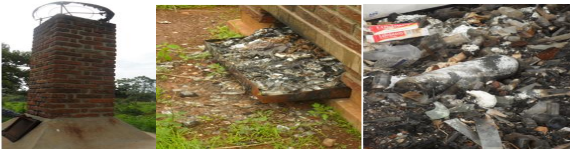
Picture Set 2. Sub-optimal healthcare waste management practice. Note that the incinerator is only two years old and is already showing signs of deterioration due to the load of waste incinerated. There is no waste minimization and segregation practices at this health care facility visited.
