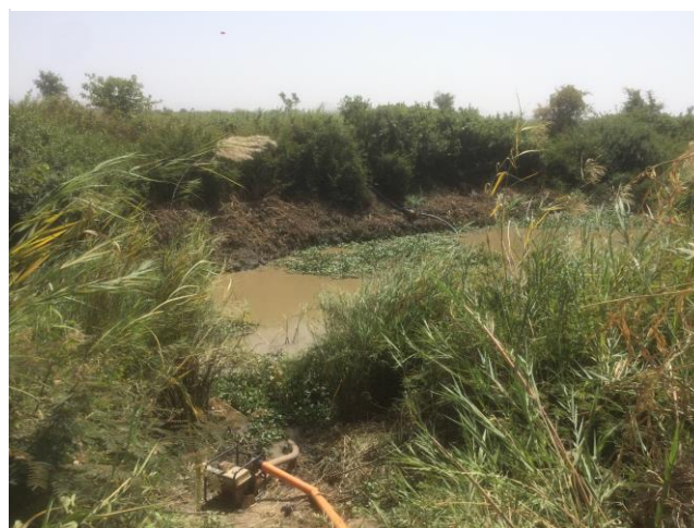
Figure 8: Pumping in a Bénoué tributary
