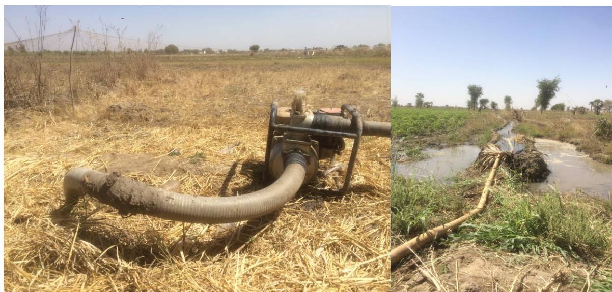
Figure 9: Manual drilling and motor pump - Earth channel in backfill with counter-slope
