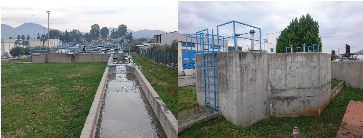
Figure I-5: Anaerobic & Anoxic Aeration Tank Line and Selector Tank
