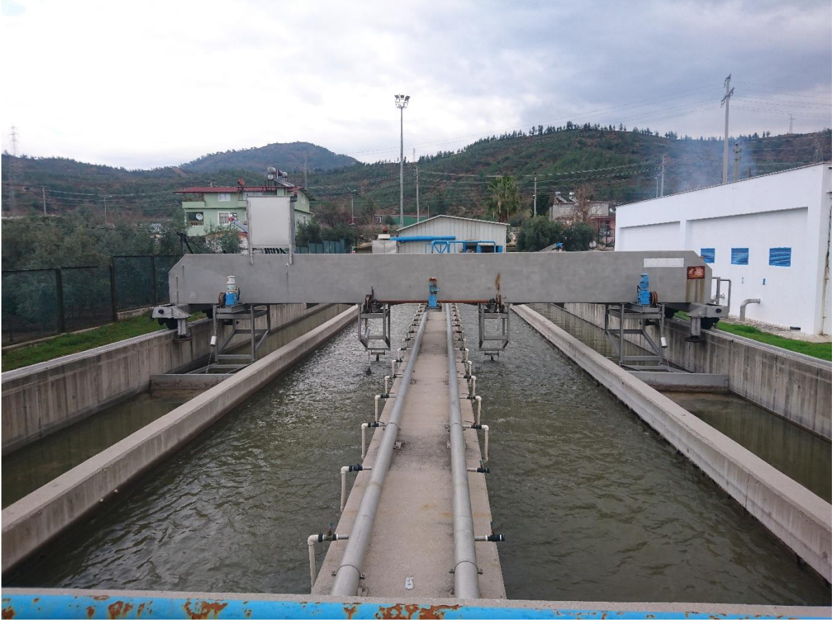
Figure I-4: Grit Chamber
