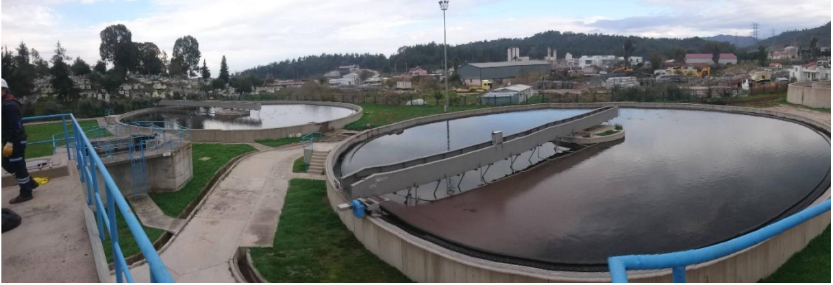
Figure I-8: Final Sedimentation Tank
