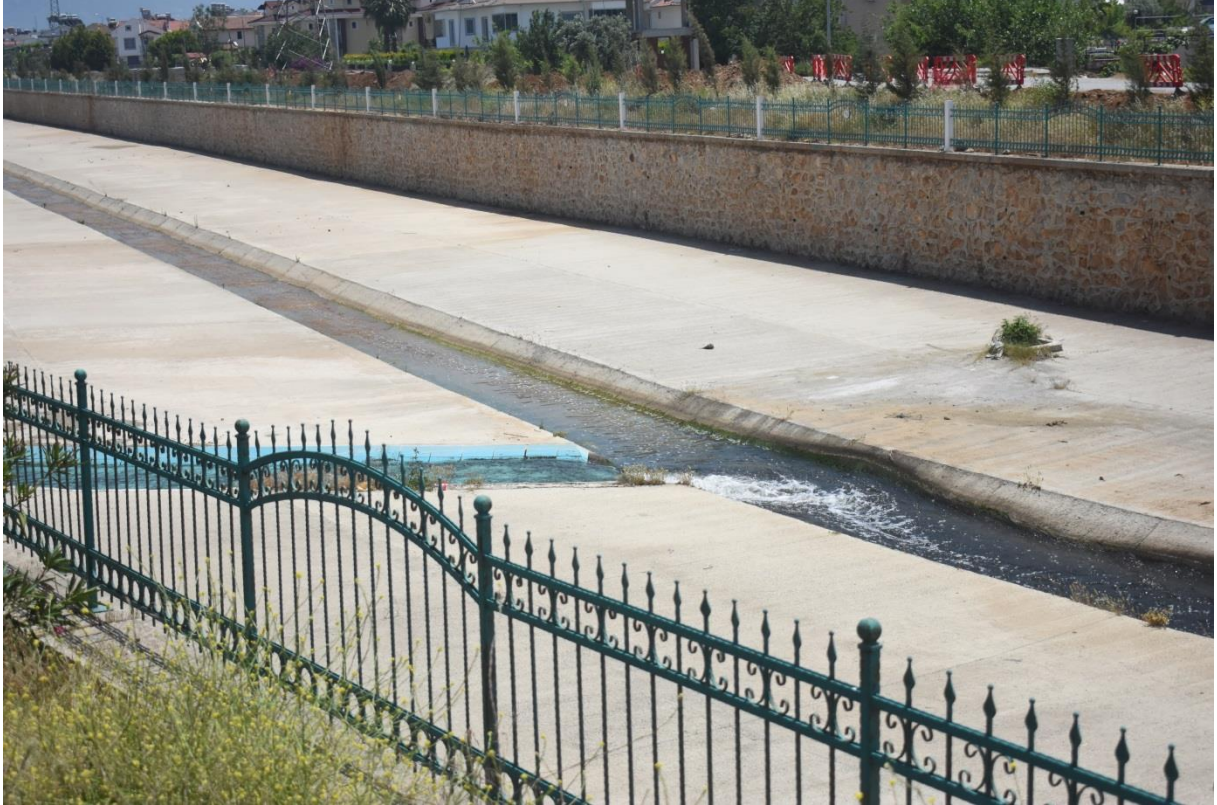
Figure V-20: Existing discharge point
