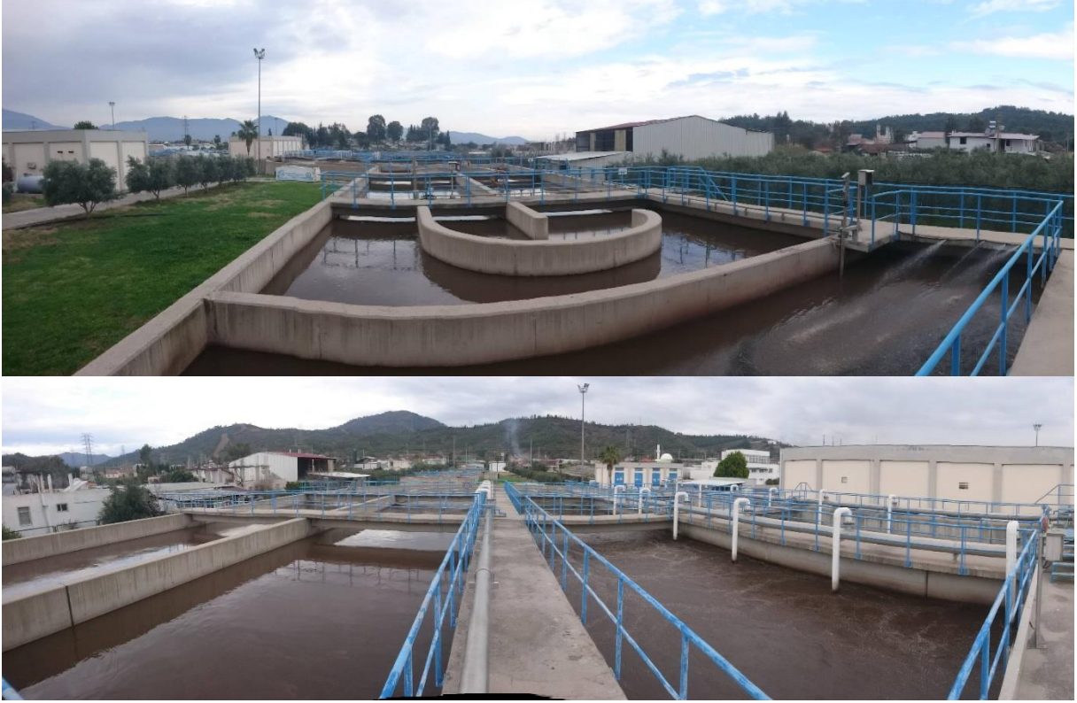
Figure I-6: Aeration Tank
