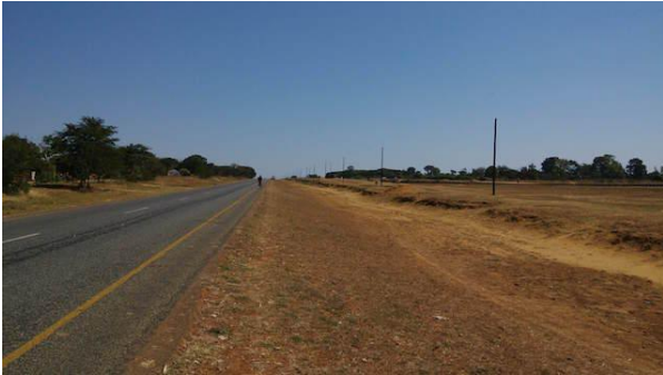
Photo 3: View of a series of poles along the M12
